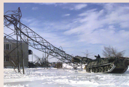
Canadian soldiers working on a toppled power transmission tower in January 1998.
